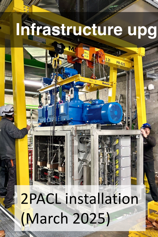
2PACL support frame in USA15 CV room
