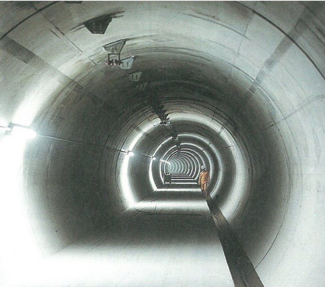
LEP tunnel before installation of bending magnets
